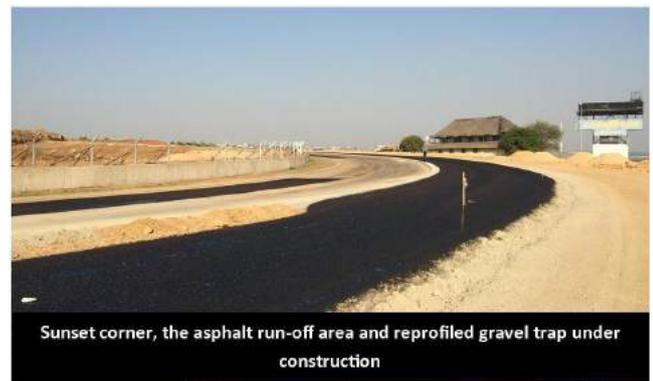
Sunset corner, the asphalt run-off area and reprofiled gravel trap under construction
