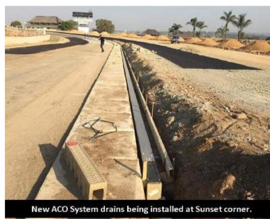
New ACO System drains being installed at Sunset corner.
