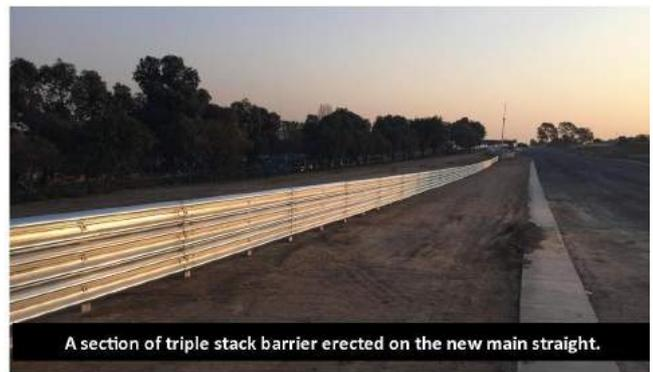
A section of triple stack barrier erected on the new main straight.
