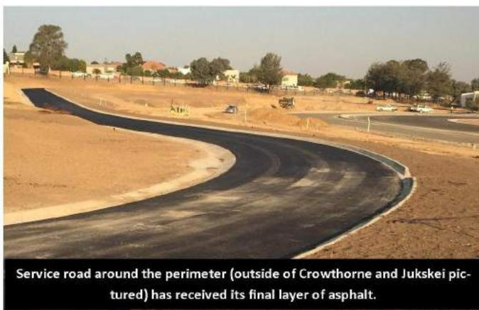
Service road around the perimeter (outside of Crowthorne and Jukskei pictured) has received its final layer of asphalt.
