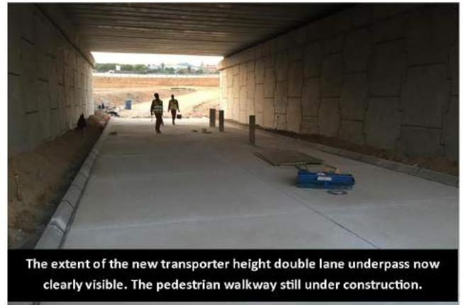
The extent of the new transporter height double lane underpass now clearly visible. The pedestrian walkway still under construction.
