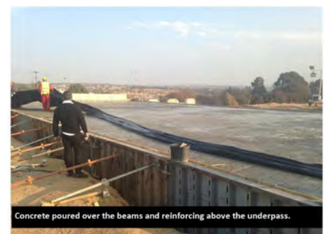
The first load of concrete is poured, 39 truck loads to follow.
