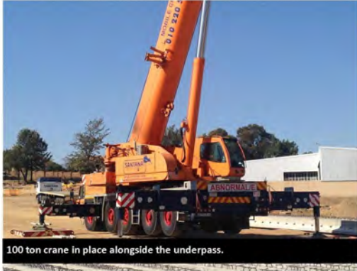
First load of beams delivered on site. The 100 ton crane in place to offload the beams alongside the underpass.
