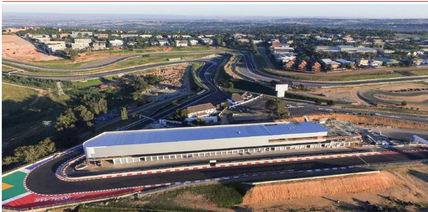
The impressive new Pit Building and International Convention Centre nearing completion.
