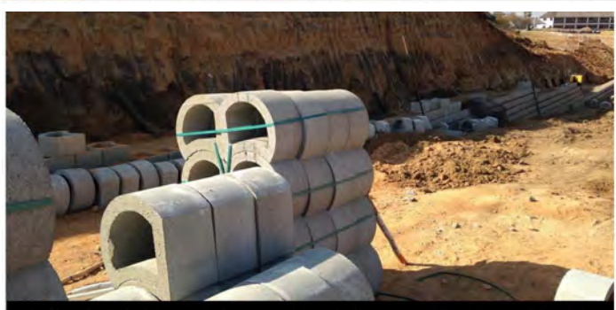
Construction of the new retaining walls at The Crocodiles has commenced.
